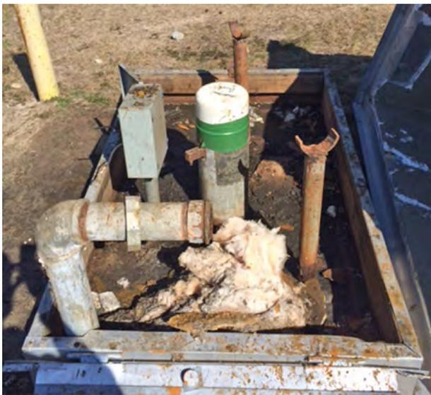
**Figure 20. Unused supply well AIK-0344 at Oakwood-Windsor Elementary School in Aiken County. The well is 404 feet deep well and is screened in the Crouch Branch aquifer.**
