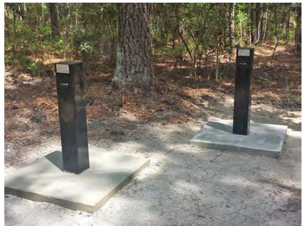
Figure 18. New monitoring wells at Hobcaw Barony in Georgetown County. GEO-0387 (left) is screened in the Gordon aquifer (95 feet deep) and GEO-0386 (right) is screened in the surficial aquifer (39 feet deep).
