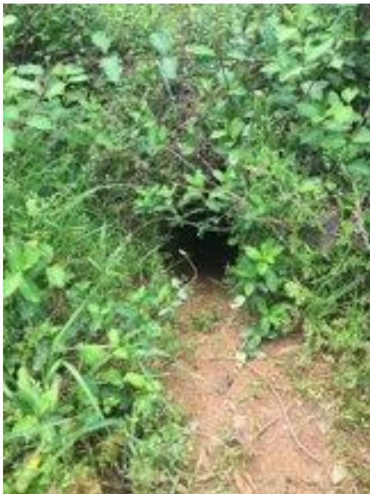
Photograph 14: Stormwater Drain from Parcel 2 into Parcel 3 wetlands
