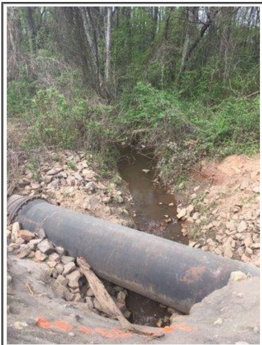
Photograph 28: Historical ditch outfall near Willard St
