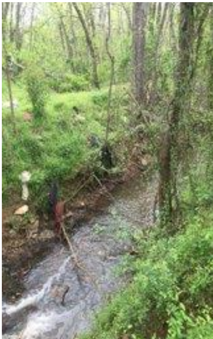
Photograph 18: Outfall from wetlands upgradient of Vaughn Landfill into wetlands downgradient of landfill
