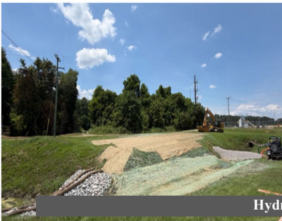
Geotextile Fabric Laid before Backfilling with 2-3 feet of New Soil
