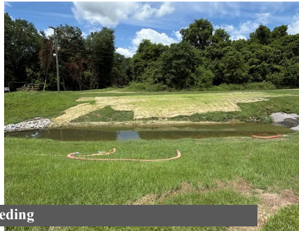
Geotextile Fabric Laid before Backfilling with 2-3 feet of New Soil
