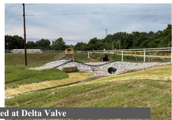
Erosion Matting Installed
