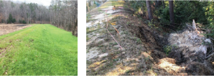
Dam Safety Staff Photo - Well Maintained Dam (left), Uprooted Trees (right)
