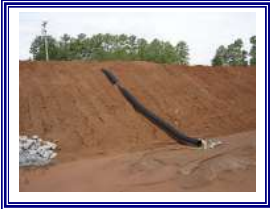
Pipe Slope Drain
