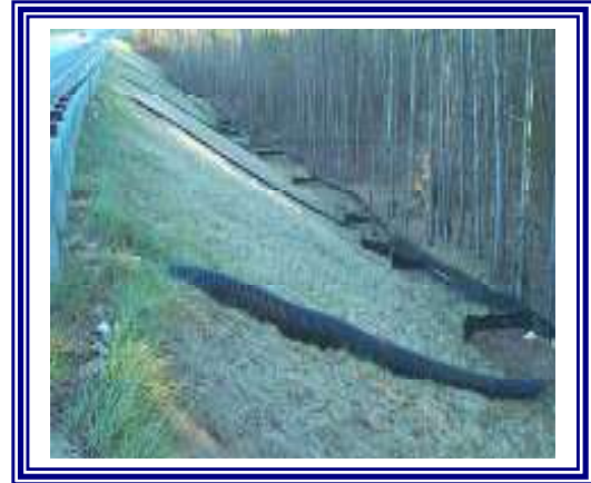
Pipe Slope Drain
