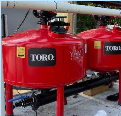
Filter Stations for Water Reuse
