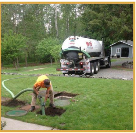
Figure 3.8 A septic system pump out (Vac-Tec Septic & Water LLC)
