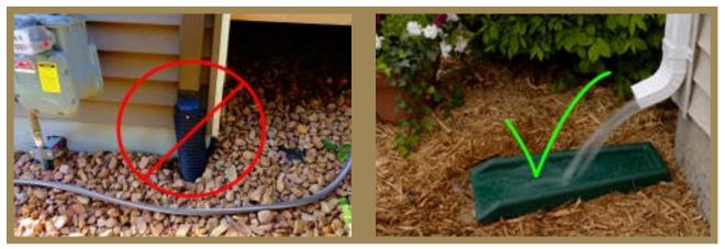
Figure 5.27 Downspout disconnect allows stormwater to recharge groundwater (The Pocket)
