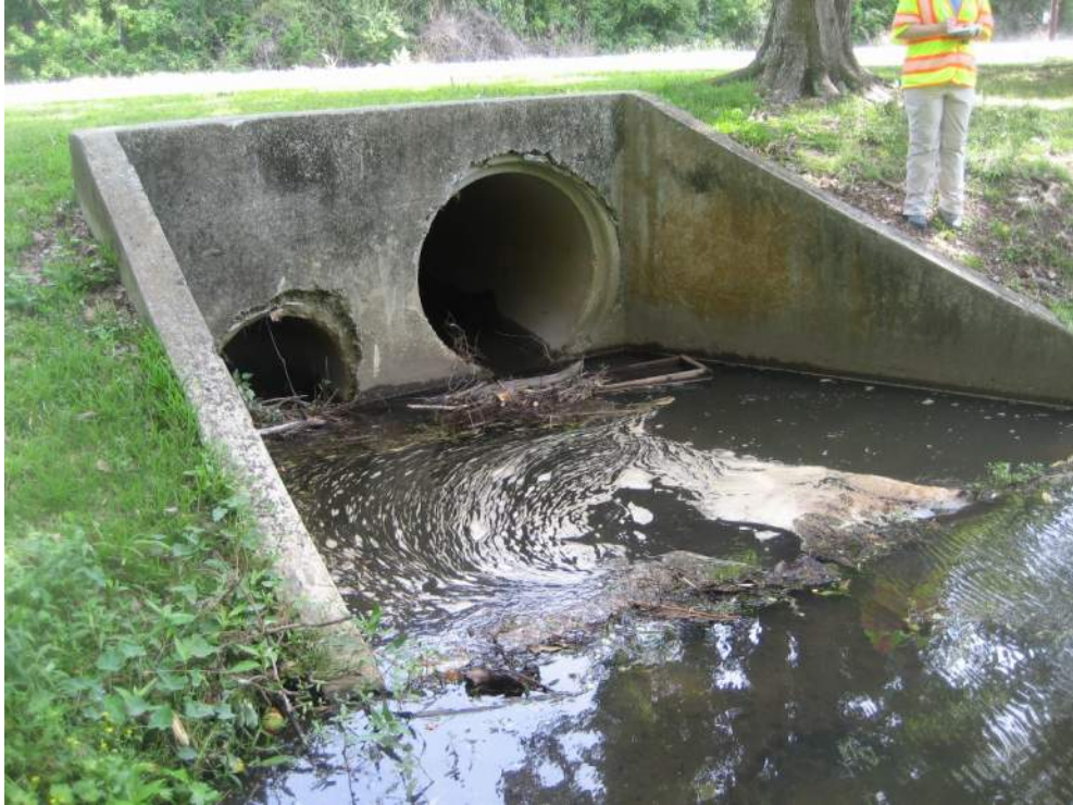
Figure 13 – Culvert Crossing under Murray Drive
