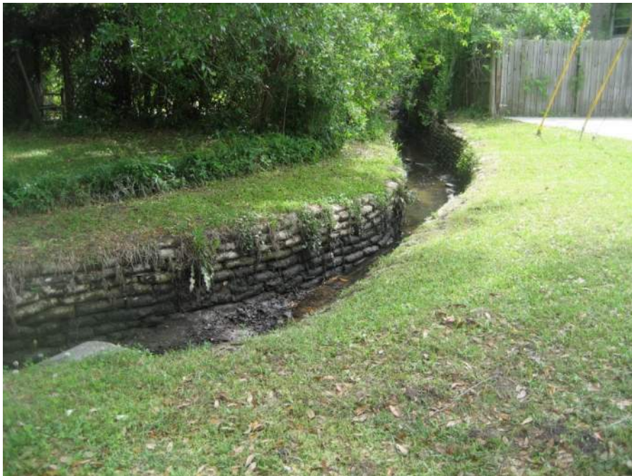
Figure 12 – Example of a concrete lined channel in a residential neighborhood that outfalls into Turkey Creek
