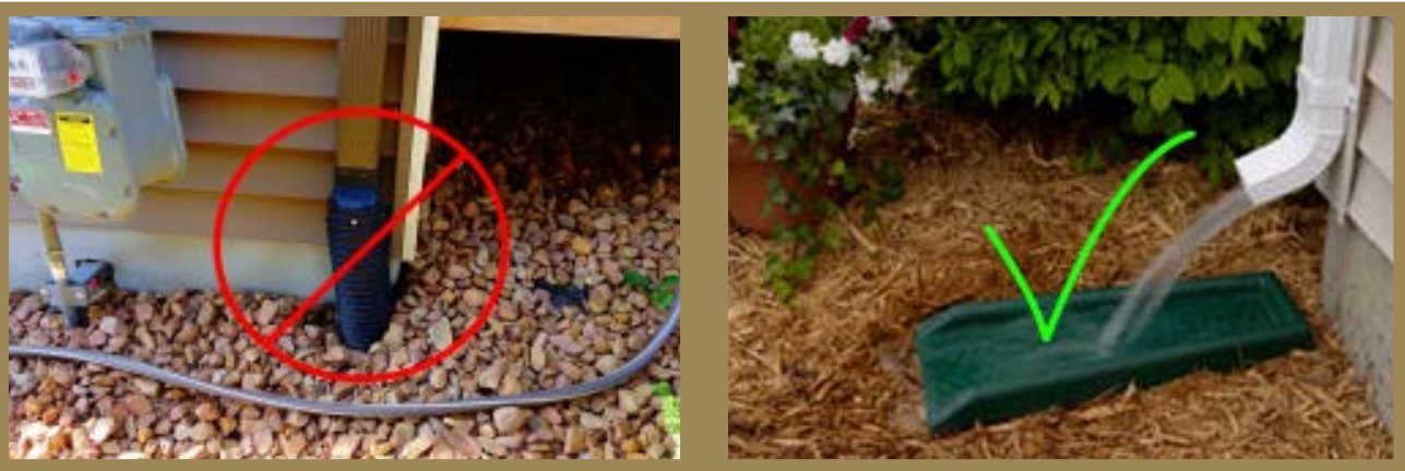
Figure 5.27 Downspout disconnect allows stormwater to recharge groundwater (The Pocket)
