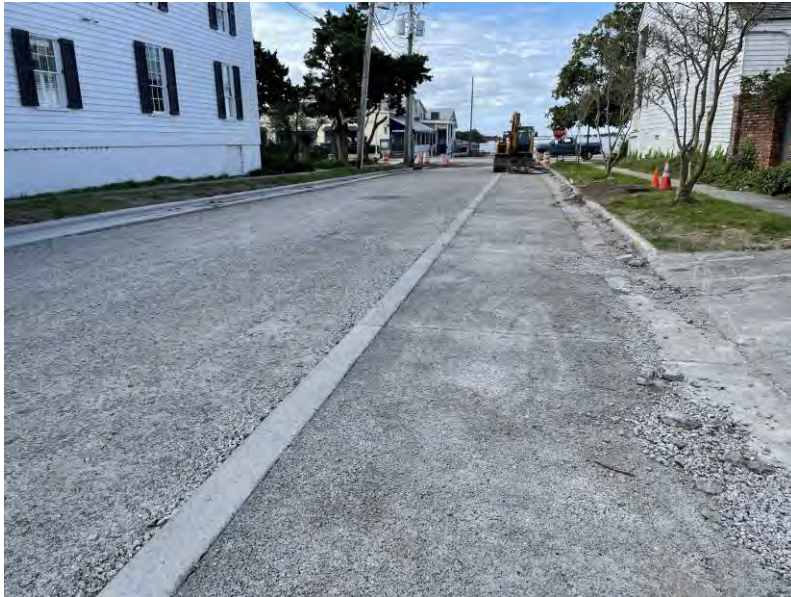
FIGURE 61: PERMEABLE PAVING INSTALLATION IN BEAUFORT, NC
