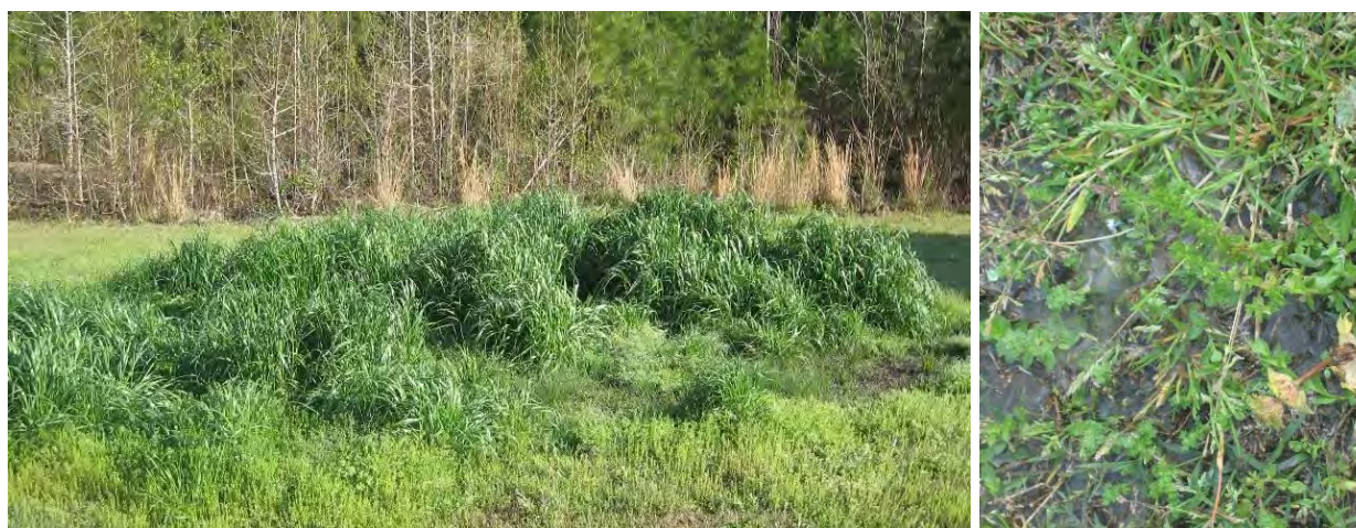
FIGURE 33. EXAMPLE FAILING SEPTIC SYSTEMS
