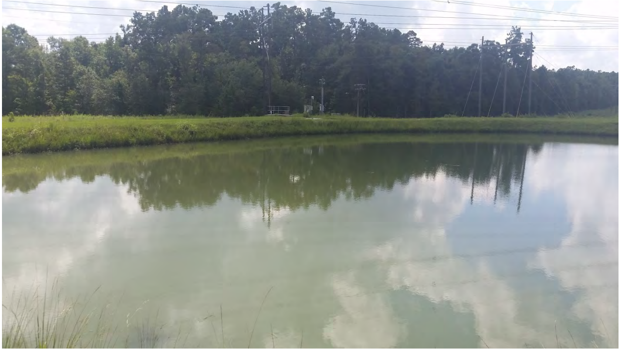
Figure 7 - Coal Pile Runoff Pond #2 (looking south)
