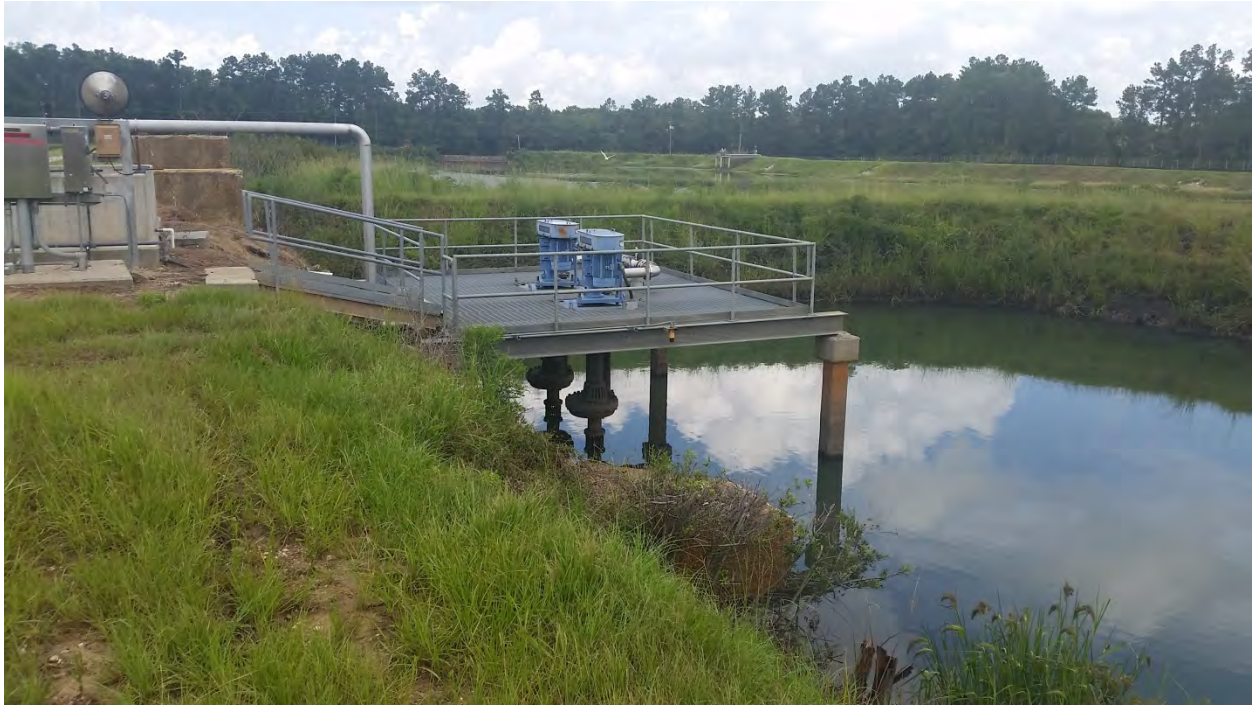
Figure 13 - Spray Pond SE Pump Station
