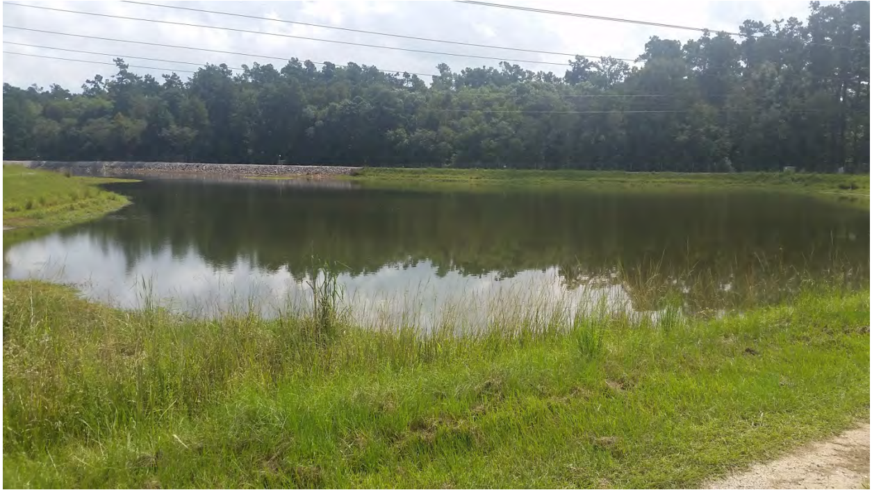
Figure 1 - Settling Pond #2 (looking NE)
