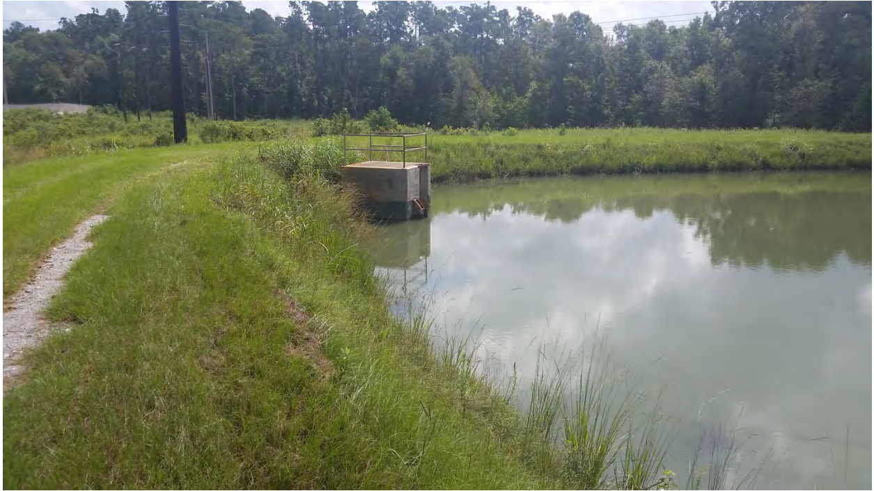
Figure 5 - Coal Pile Runoff Pond #2 (looking east)
