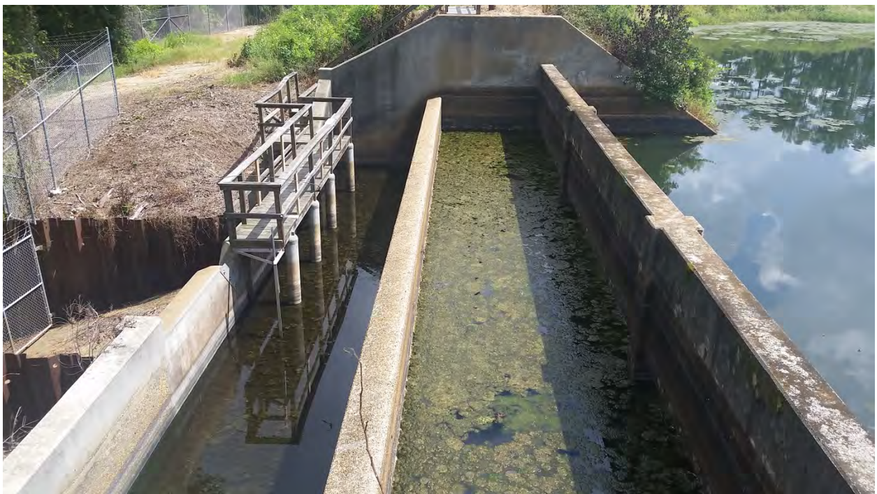
Figure 14 - Spray Pond Outlet Structure
