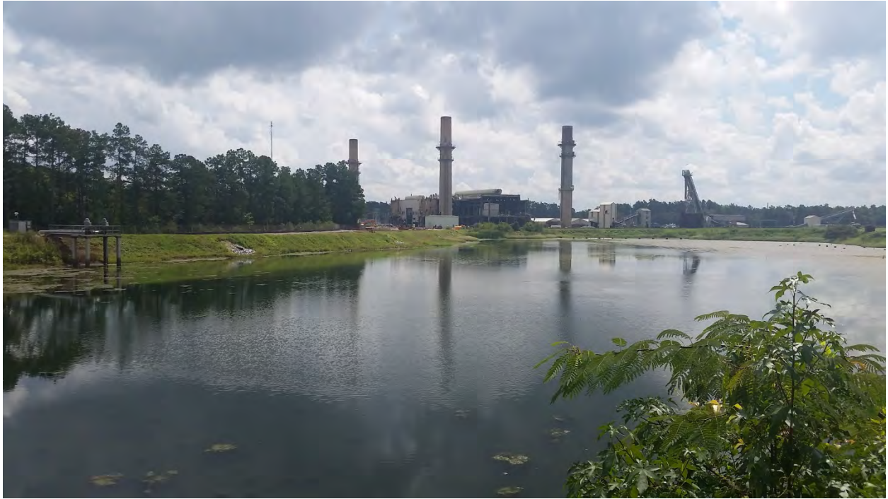
Figure 15 - Spray Pond (looking ESE)
