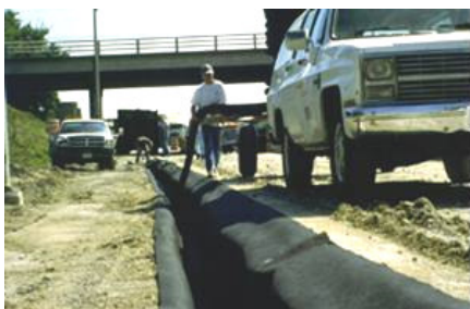
Subsurface Drain
