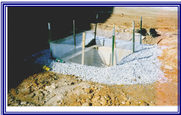
Hardware Fabric and Stone Inlet Protection
