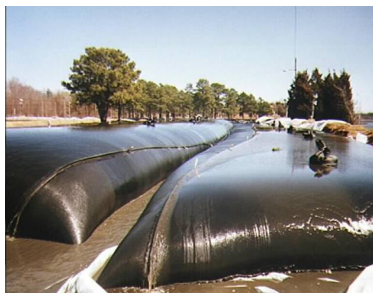
Construction Dewatering
