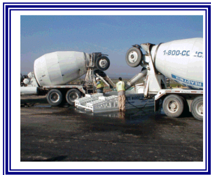
Concrete Truck Washout
