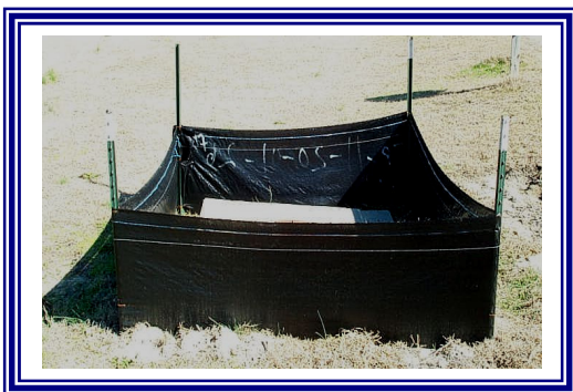
Filter Fabric Inlet Protection
