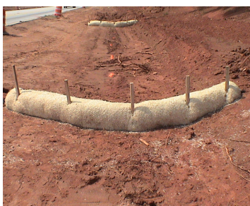
Sediment Tube Check Dam
