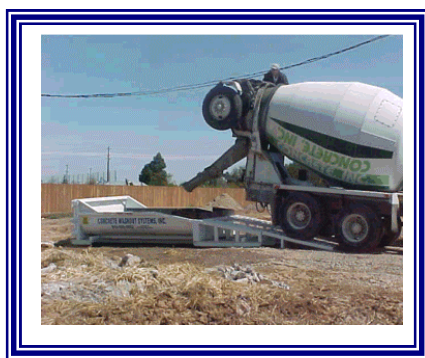
Concrete Truck Washout
