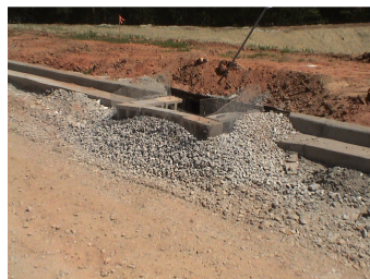
Block and Gravel Inlet Protection
