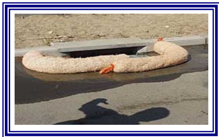
Weighted Inlet Tube
