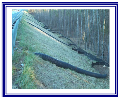
Pipe Slope Drains
