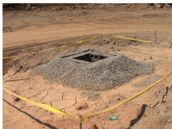
Block and Gravel Inlet Protection
