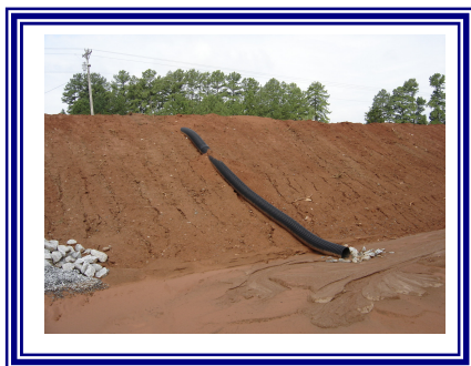
Pipe Slope Drains
