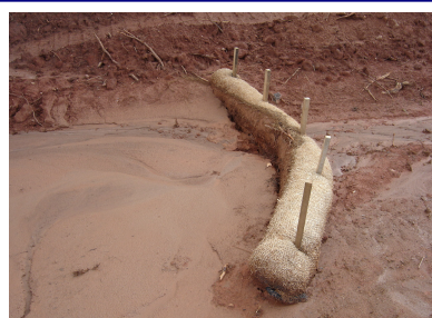
Sediment Tube Check Dam
