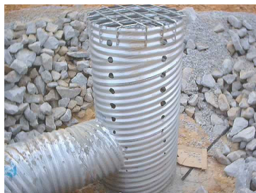
Sediment Basin Perforated Riser
