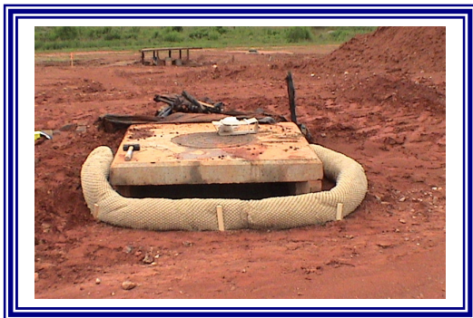
Sediment Tube Inlet Protection
