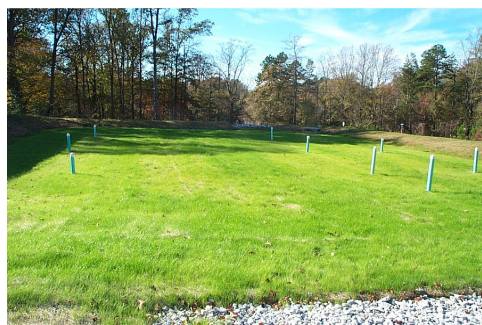
Bioretention Area with un-cut clean outs
