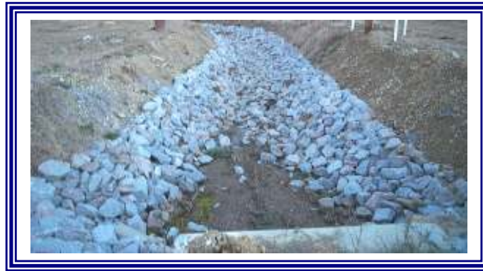
Riprap Lined Channel
