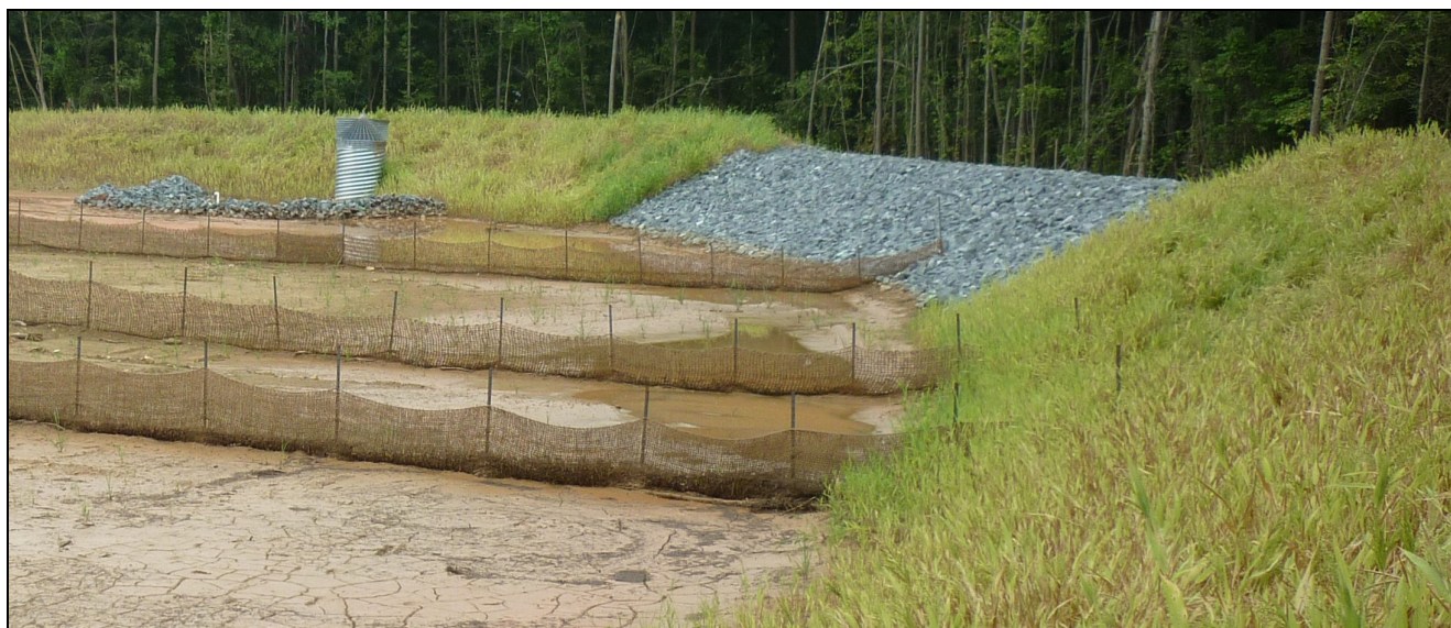
Photo: Porous Baffles
