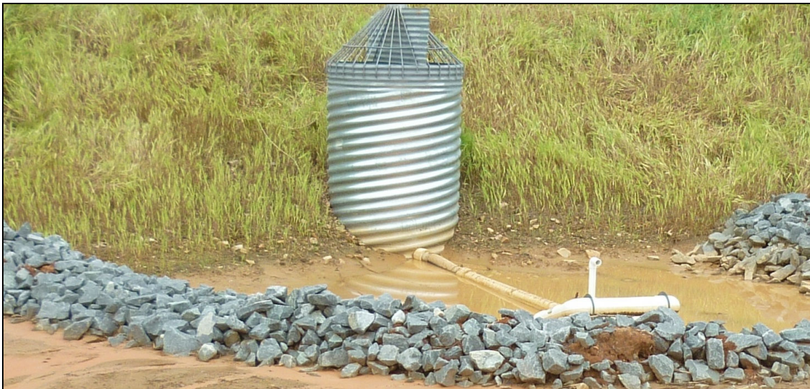
Photo: Principle Spillway's Riser Structure with Skimmer
