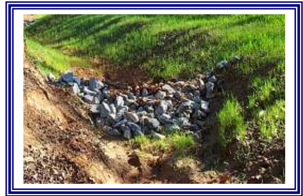
Rock Check Dam
