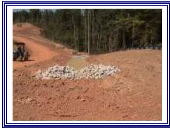
Rock Check Dam
