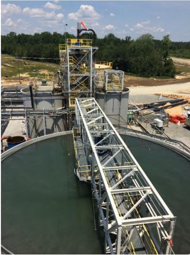
**Figure A-54 Tails Thickener and Cyanide Destruct Circuit**
