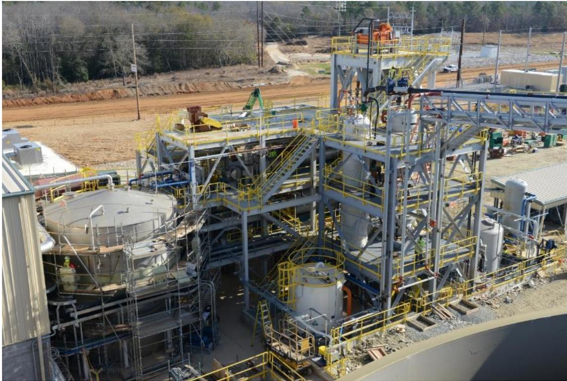
**Figure A-52 Elution Circuit – Acid Wash, Barren Tank, and Carbon Regeneration Rotary Kiln**
