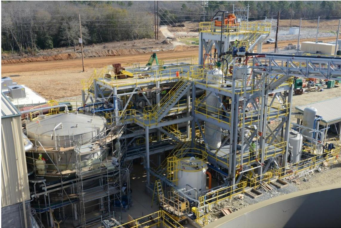
**Figure A-54 Elution Circuit – Acid Wash, Barren Tank, and Carbon Regeneration Rotary Kiln**
