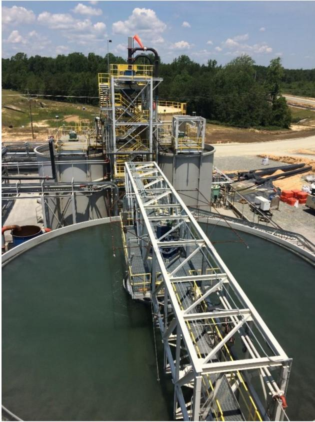
**Figure A-56 Tails Thickener and Cyanide Destruct Circuit**
