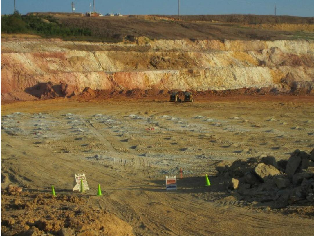
**Figure A-11 Drill Holes in a Blast Pattern**
