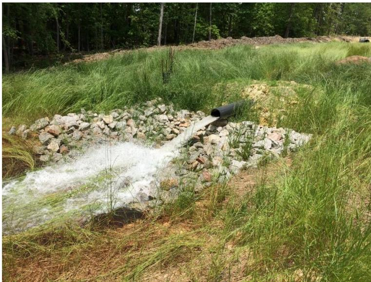
**Figure A-74 NPDES 003 Outfall for Water Treatment Discharge**
