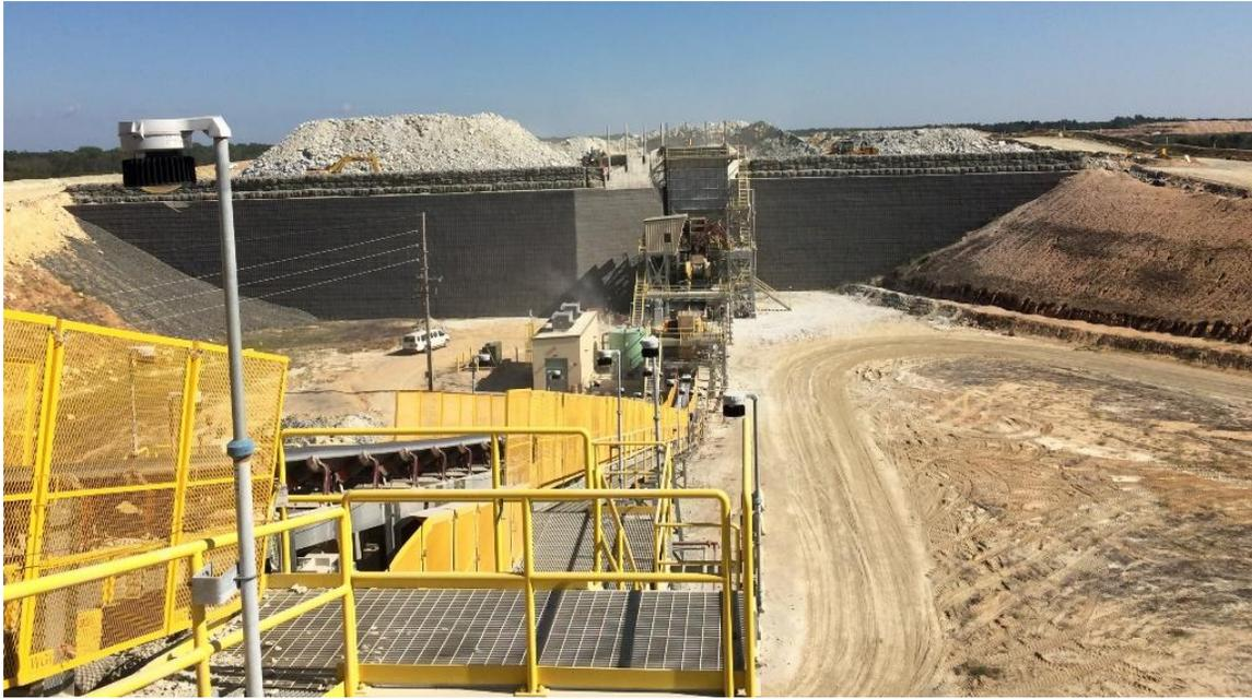
**Figure A-45 Run-of Mine Pad and Crushing Circuit**
